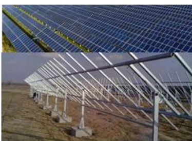
Solar Panel Bracket Hot-Dip Zn-Al-Mg Coated Steel
