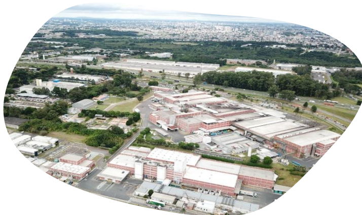
Figure 1 - Curitiba Plant Mondelez Brazil
