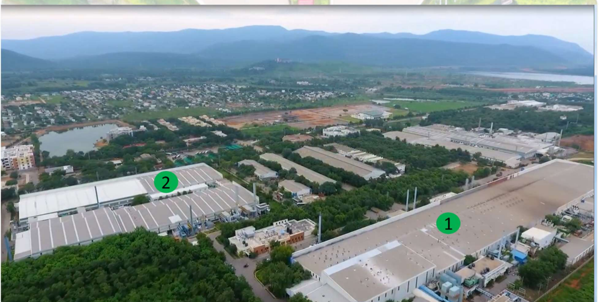
1 4 Wheeler Battery manufacturing facility
